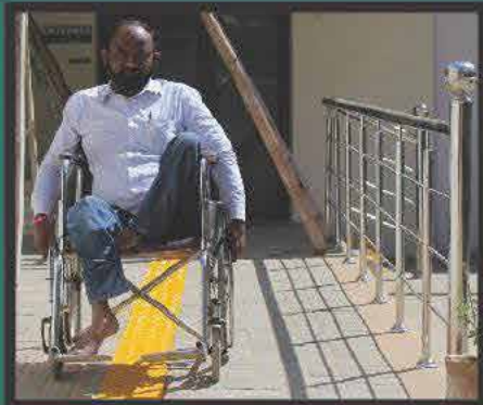
Ramps at a ratio of 1:16 which can be accessed by persons with physical impairments
