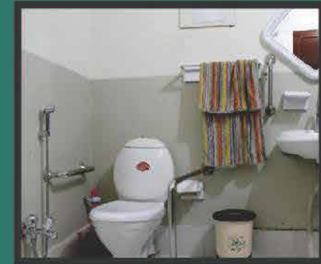
Accessible bathrooms for persons with disabilities
