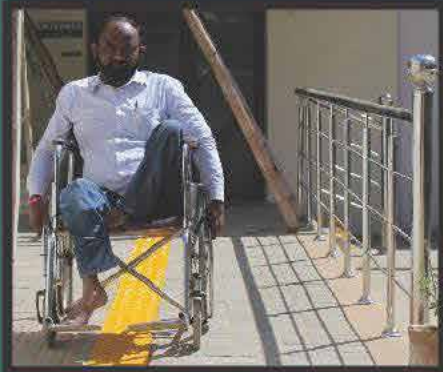
Ramps at a ratio of 1:16 which can be accessed by persons with physical impairments
